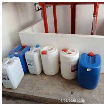
NC No secondary Containment diesel containers.jpg
